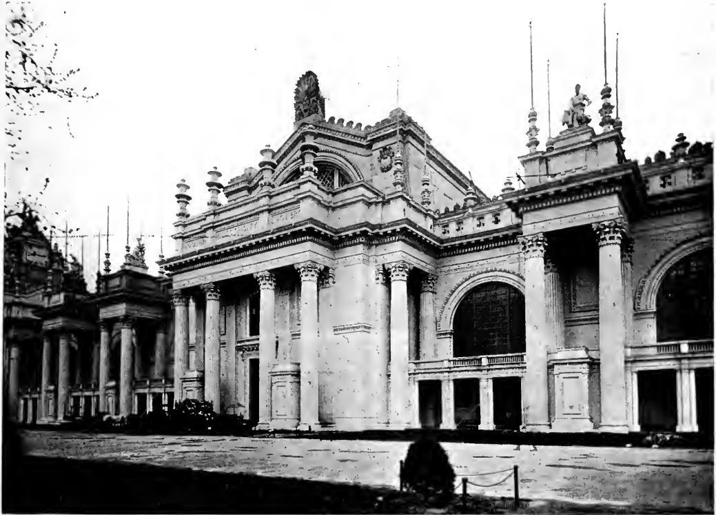
FIG. 19.—ENTRANCE TO ELECTRICITY BUILDING.
